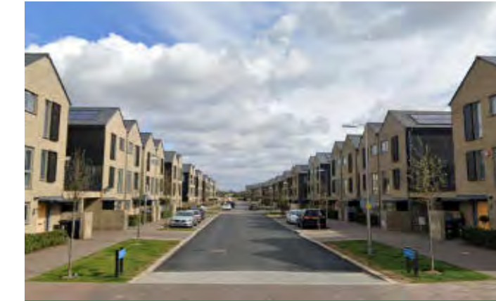
New Hall (phase 2) achieves a consistent and strong street character, with a mirrored architectural style down both sides and a sense of enclosure.
