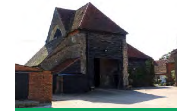
LATTON PRIORY FARM INCLUDES HERITAGE ASSETS
