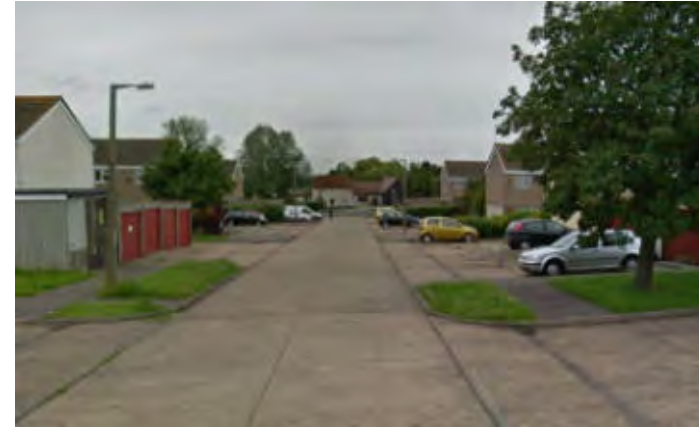
South Harlow has a number of row house blocks, with garages on the end. This creates a dead street frontage and a lack of surveillance.
